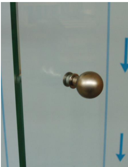
Screw the door handle from the Inside and outside with a shim.
